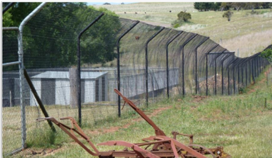
Regulation 6ft chain mesh fence with overhang
